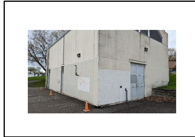
Photograph 2: Exterior view of Sewage Pumping Station, southeast corner.
