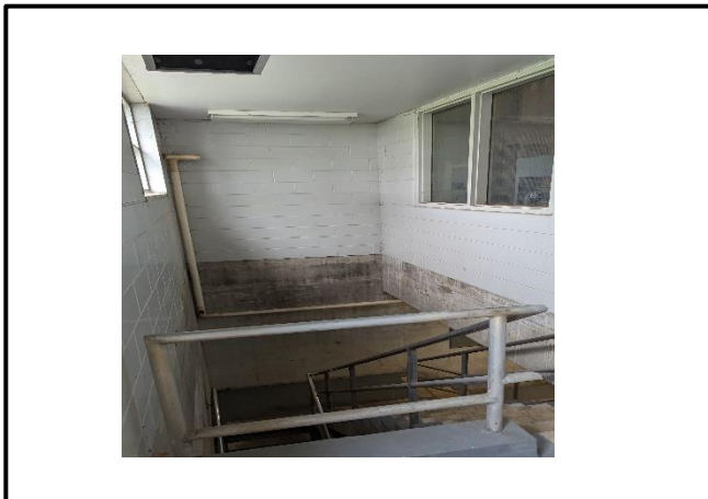
Photograph 3: View of Loc 1, entrance vestibule and stairwell.
