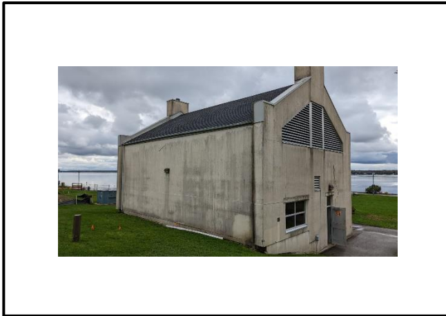
Photograph 1: Exterior view of Sewage Pumping Station, northwest corner.
