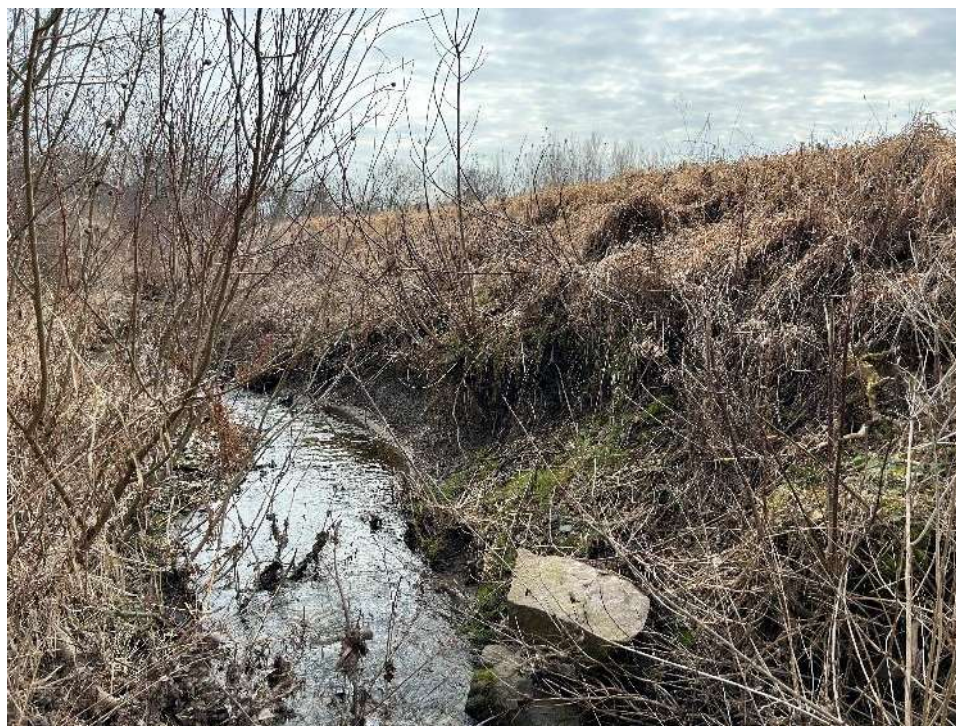
Photo 2 Viewing west along Arena Creek bed. North berm visible on right side. Evidence of toe erosion can be seen.
